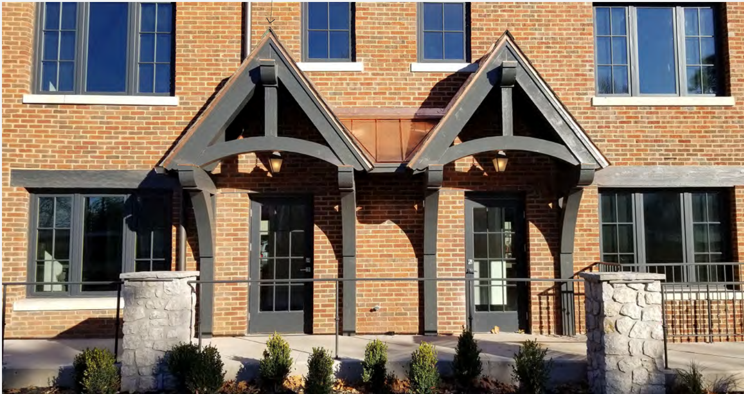
new canopy entrance clad in a slate and copper roofing
